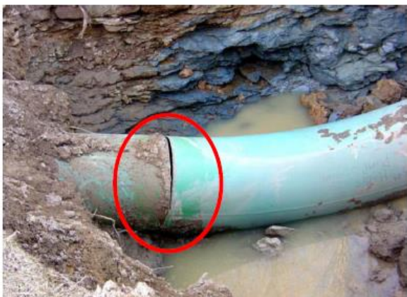
Figure 28 Connection of different pipeline section with different shape and wall thickness [54]
